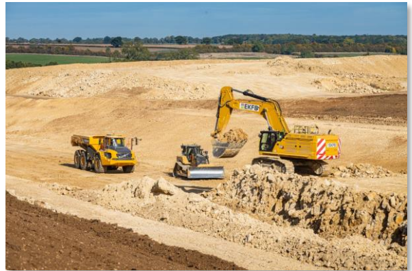
Figure 7: Plant carrying out excavation works at the Turweston Cutting, Autumn 2022.
