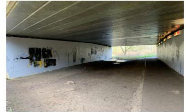
The existing traffic-free route is already well used but is unsurfaced making it very muddy. A sealed surface would ensure it can be used all year-round. The path at the A43 underbridge should be widened to make it more comfortable. Community artwork protected with an anti-graffiti coating could be commissioned to deter anti-social behaviour
