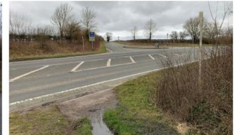
Crossing point not currently provided for over the A422
