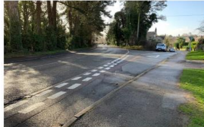
Very wide junction radii and steep gradient makes it very difficult for pedestrians to navigate along Northampton Road and creates a hooking risk for cyclists in the carriageway. The footway ends at Burwell Hill forcing pedestrians to cross the road with no facility or go an indirect route
