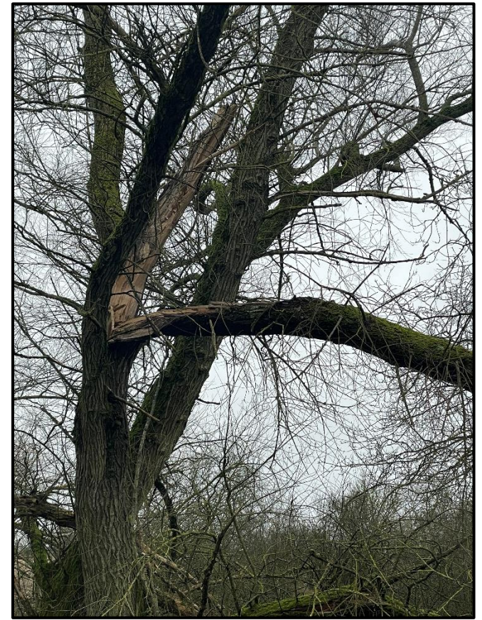
Figure 3: a view of the failed limb on T9
