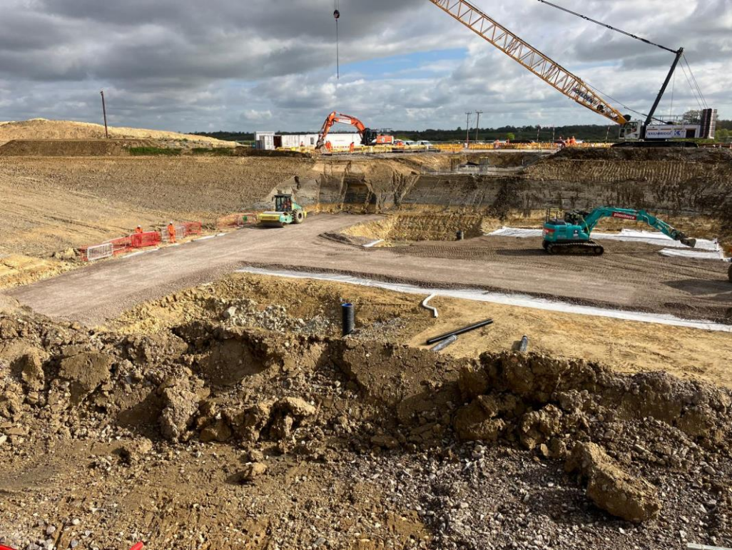
AX18 Piling complete – Preparation for the concrete
