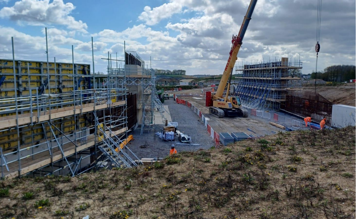
Wing Wall construction
