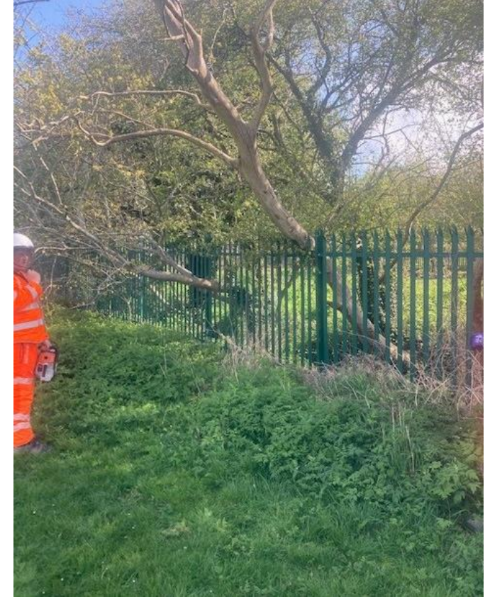
Removal of fallen trees
