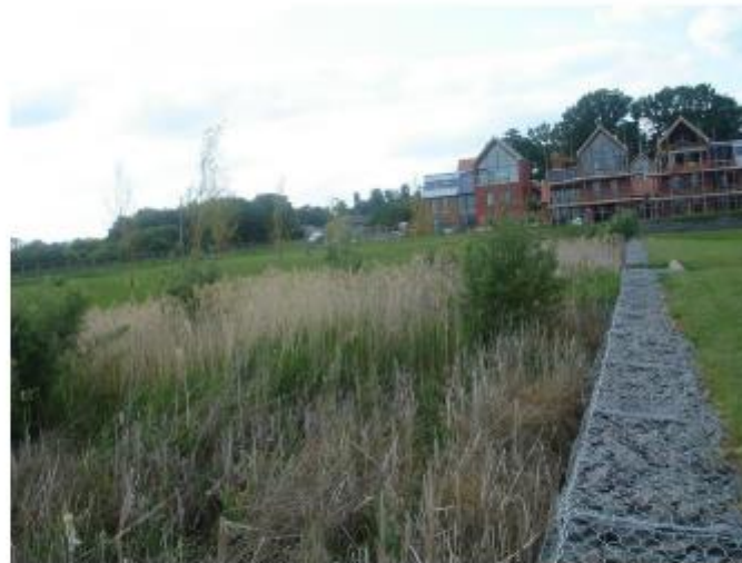
Sustainable Urban Drainage Systems: [SUDS] at Upton, Northampton
