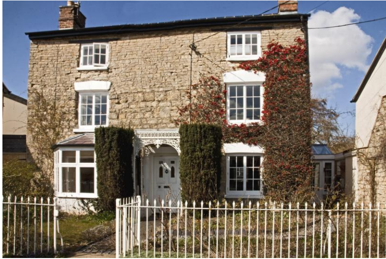
Example of a period house in High Street
